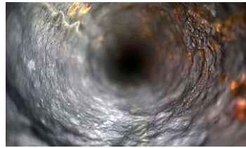
Real life problem 2 Corrosion of Piping
