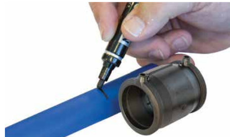
4. Witness mark correct insertion depth.
